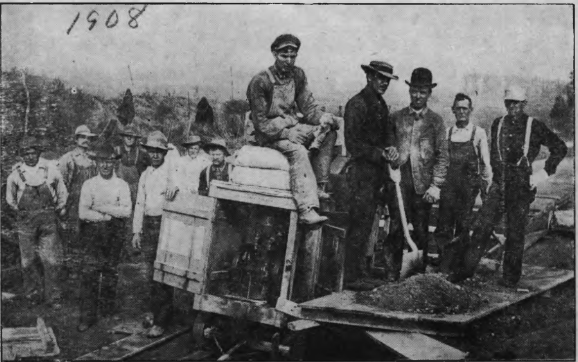
S. P. Crosson and his crew as they built the first concrete rural highway in Iowa in 1908
